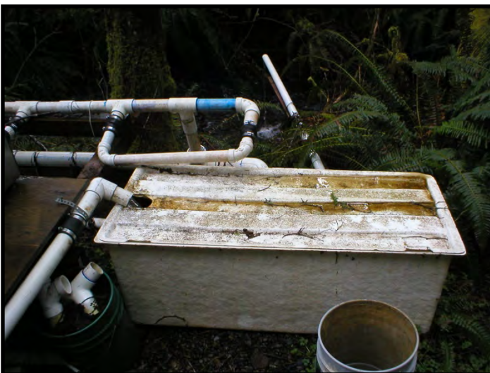
Settling tank for water discharged from the hatchboxes.
