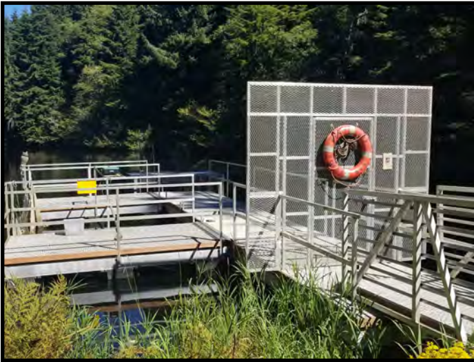
Access walkway is on the right and floating docks on either side of the net pen are shown on the left.
